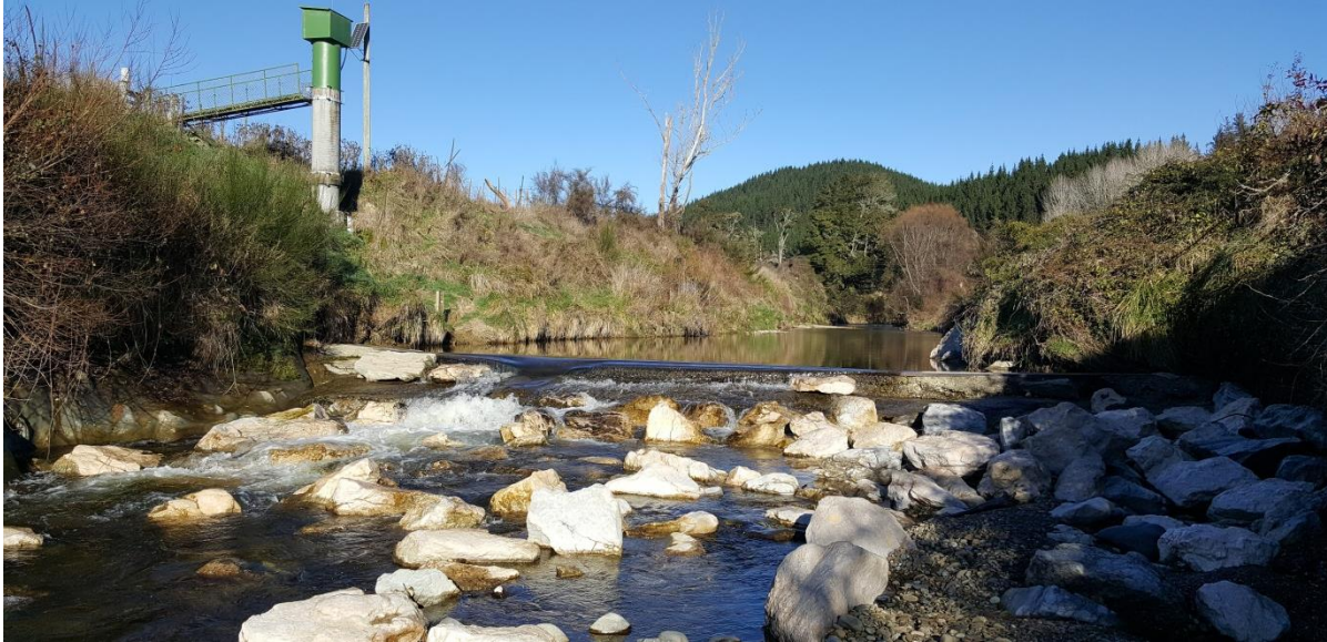
Tadmor gauging weir
