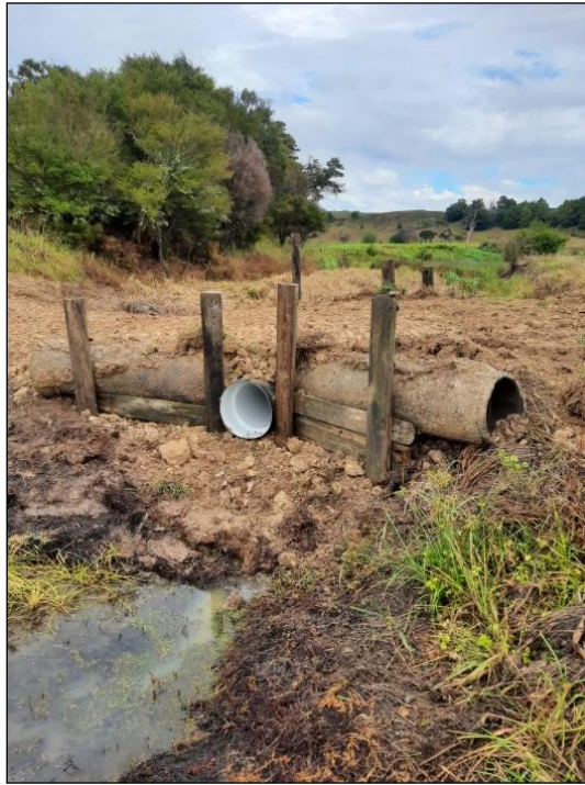
New culvert pipe at the North Pond, Jack Bisset Wetlands
