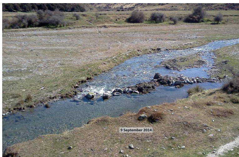
Figure 1. Glendhu Station's earth and rock barrier on the Fern Burn stream used to divert water into its water race (on right).
