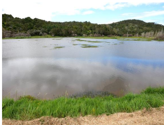
Stage 2 of Underwood Wetland development taking shape
