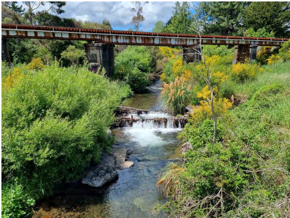
Photo 17. Mangateitei Stream (Site 11) showing the rail bridge bed control structure.
