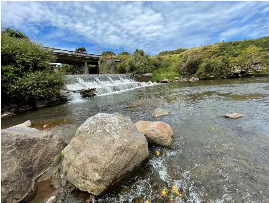
Photo 13. The 4.5m concrete diversion weir for the Opunake hydro scheme in the Waiaua River.
