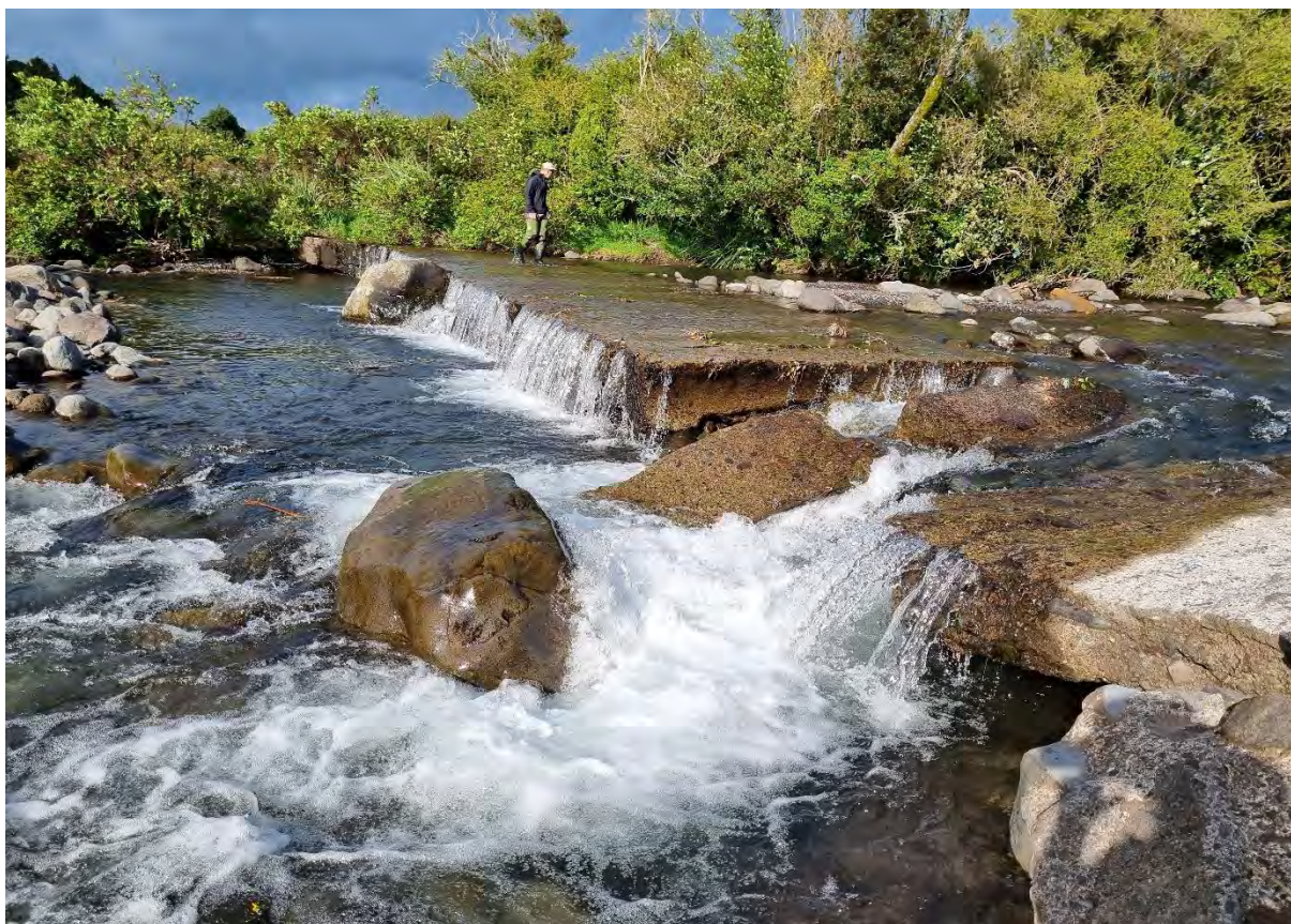
Photo 1. Disused farm access ford located in Kapuni Stream 150m downstream of Opunake Road that is an impediment to fish passage.
