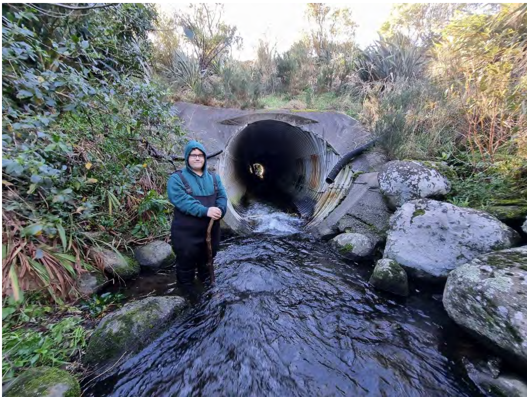
Photo 3. Wyatt Dobbin at the upstream end of the Mangamahoe Stream SH3 road culvert.
