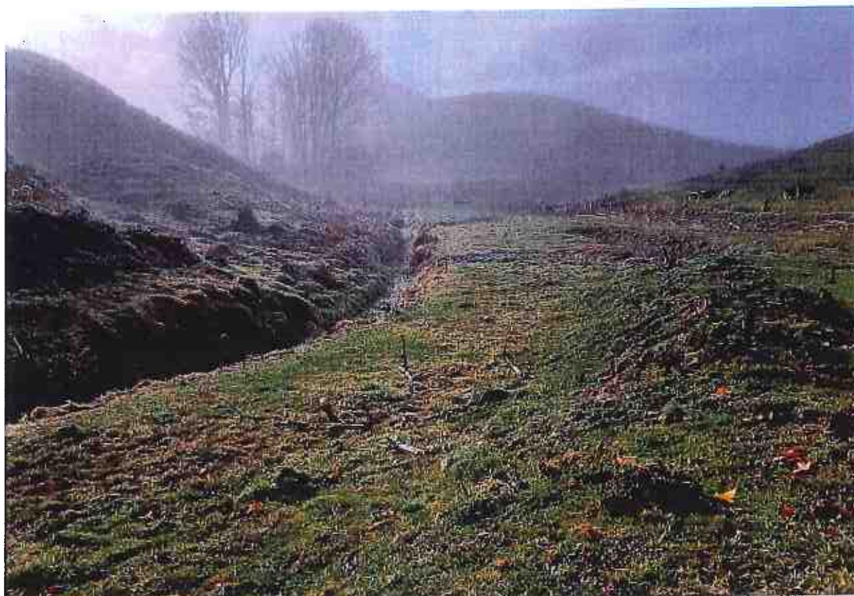
Photo 1. Dam site looking upstream
